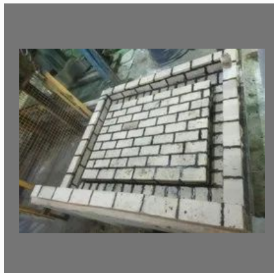
Acid Proof Brick Lining Work Pump Foundation
