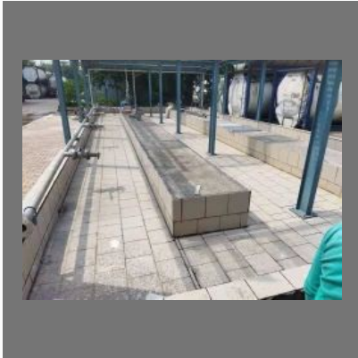
Acid Proof Tiles Lining Work
