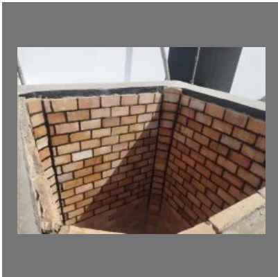
Acid proof brick lining work
