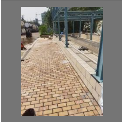
Acid Tiles Lining Work
