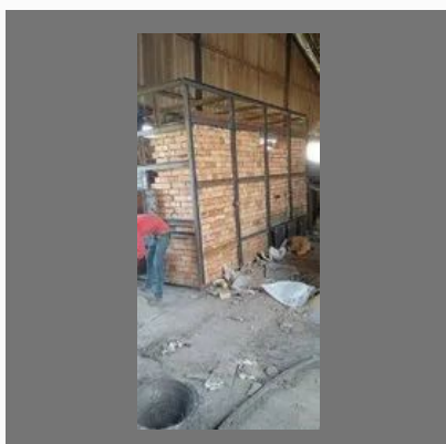
Refractory Lining work
