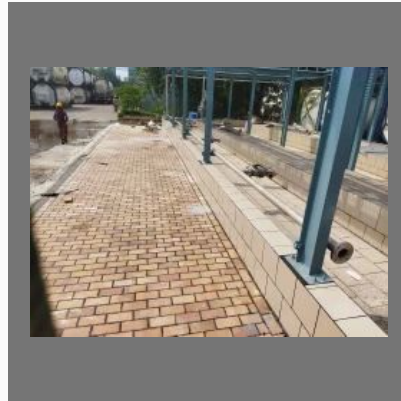
A.R. Tiles lining Work
